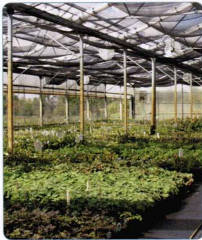
Side walls are opened and closed based on soil temperature.
